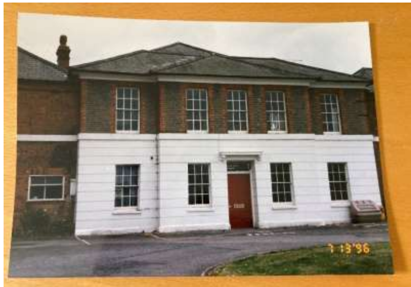
Sandleford Hospital in 1996, originally Newbury Workhouse Photo of Sandleford hospital courtesy of Val Pollitt
